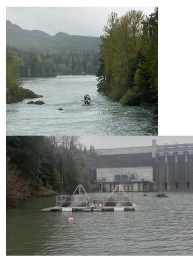
Figure H-12. Lookout Dam Tailrace – Powerhouse Channel in the old orientation where one trap was staggered behind the other (top) and in the new orientation side by side (bottom).
